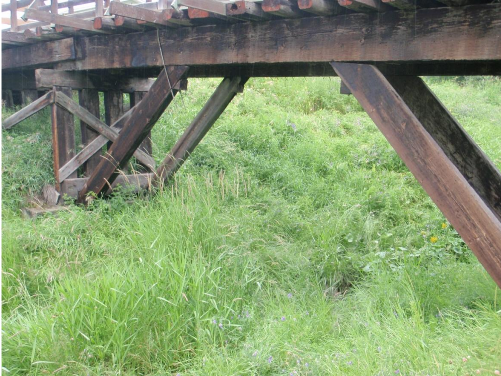
Photograph 3. Downstream side of bridge crossing, looking upstream.
