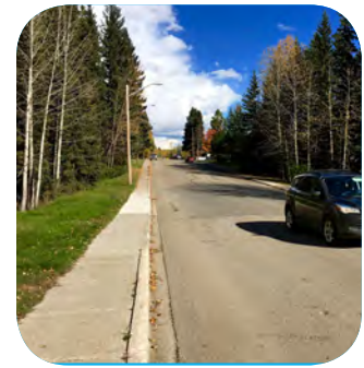
Existing 6th Ave. Streetscape
