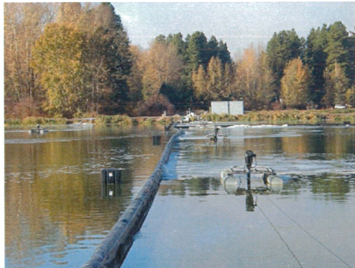
Figure 6.3 Floating Baffle Curtain and Surface Mount Aerators.
