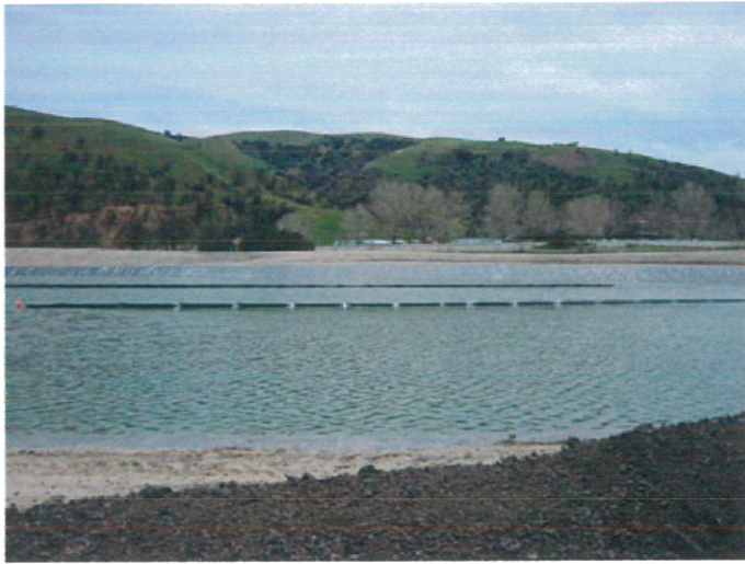
Figure 6.3 Floating Baffle Curtain and Surface Mount Aerators.
