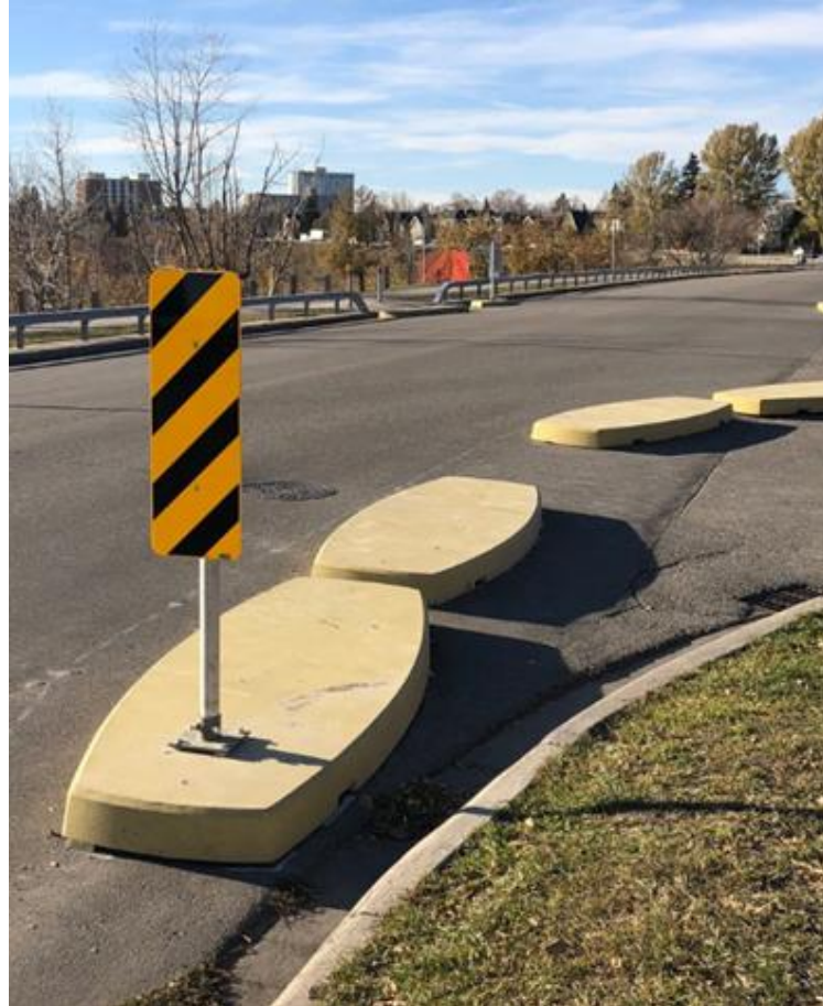
Curb extension with traffic calming blocks, Calgary (Source: City of Calgary)
